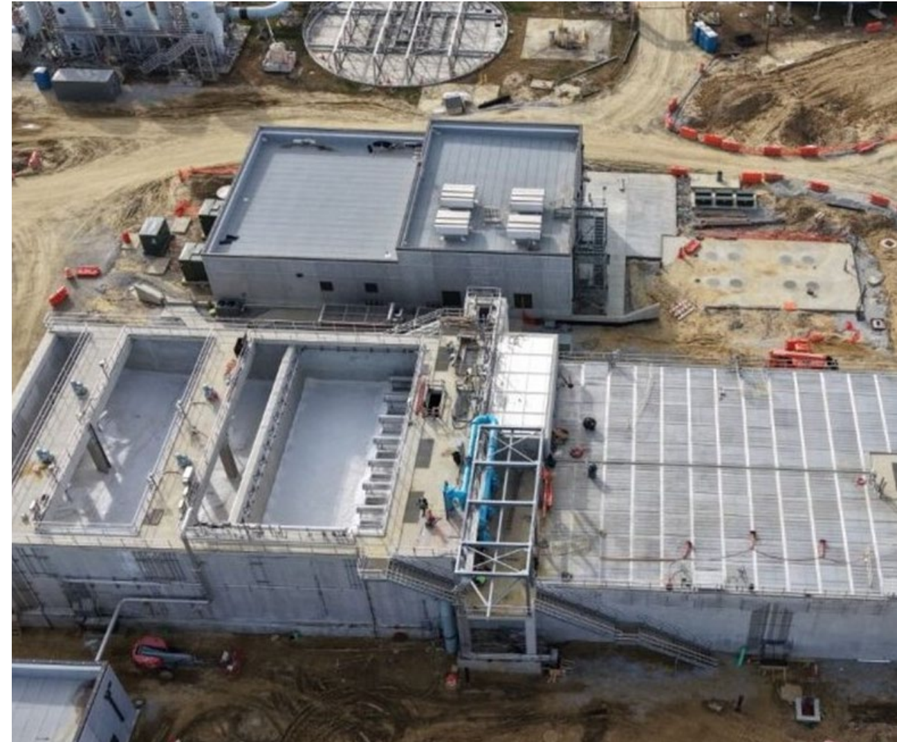
Installation and wet testing of MBBR media
